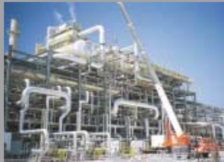
Utilities & Tanks for EQUATE
