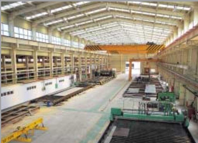
Steel Box Fabrication Line
